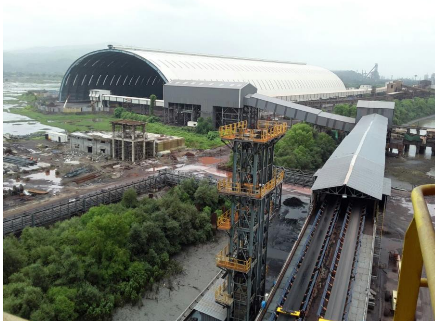
JETTY CONVEYOR INTERFACING WITH THE COVERED STORAGE FOR RAW MATERIAL (by others) OF THE STEEL PLANT
