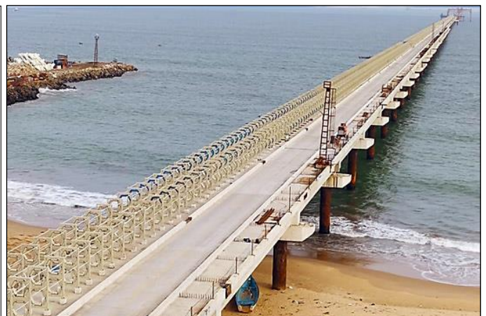
APPROACH TRESTLE CONNECTING SHORE LINE AND JETTY (9.5 KM AWAY) (Grafix is involved in MHS and interfacing)
